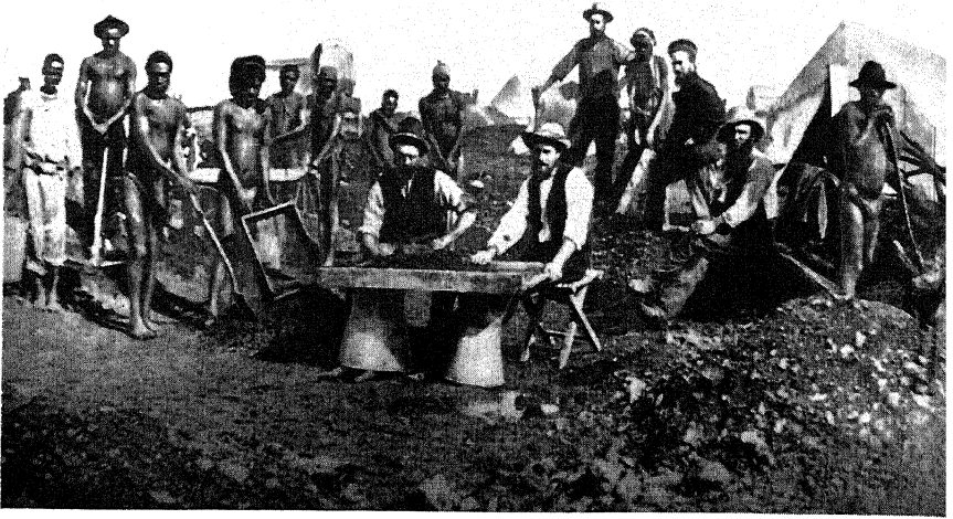
Dry sorting for diamonds in 1872 before the advent of the Hand Washing Machine Note the sorting table in the foreground
