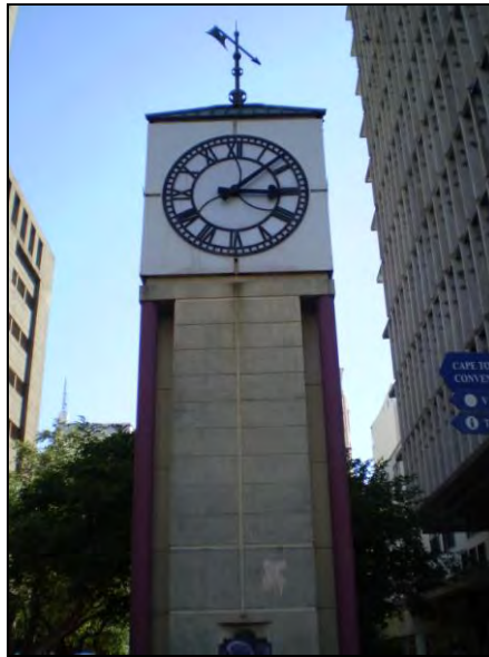
Photograph 2.B 18(a): Colonial Mutual Building Clock (upper portion and clock) 2009 O'Donoghue
